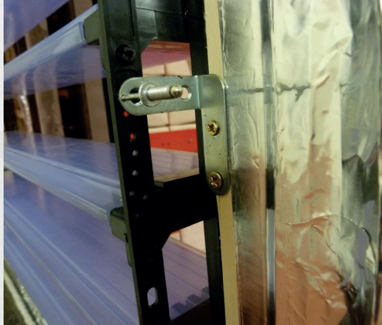
Photo 5: System for maintaining the opening angle of the blades
